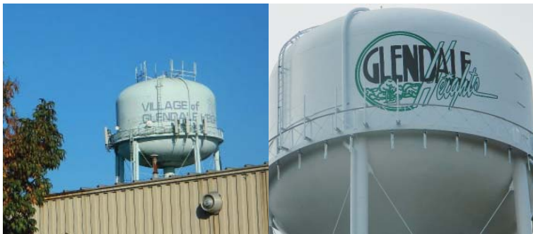
Before and after of the 1666 Glen Ellyn Road Water Tower
