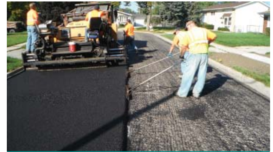
In-house Road Program on Glengary Drive, Altgeld Avenue and Scott Street
