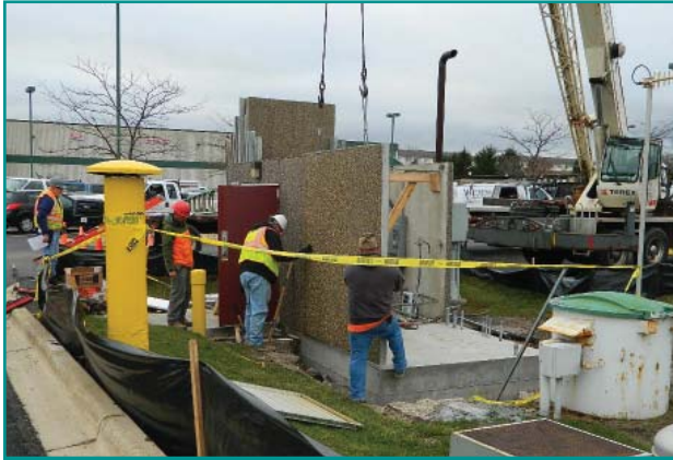
Lift Station Retrofit at 521 North Avenue
