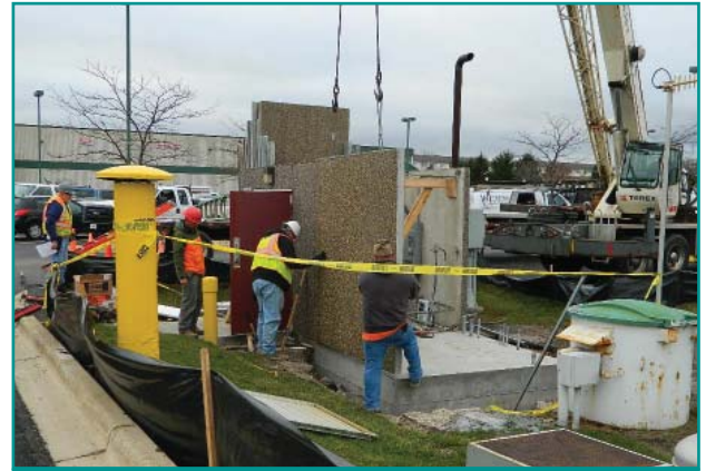
Lift Station Retrofit at 521 North Avenue
