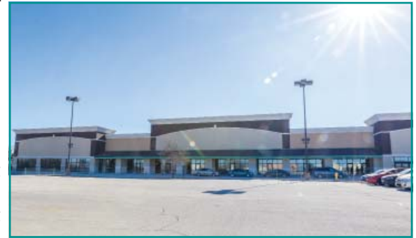
Former Dominick's is being remodeled for additional retail and storage
