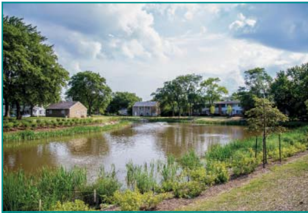
The North Ave Flood Alleviation Project alleviates flooding issues for residents surrounding James Court Pond and the Glendale Square Shopping Center
