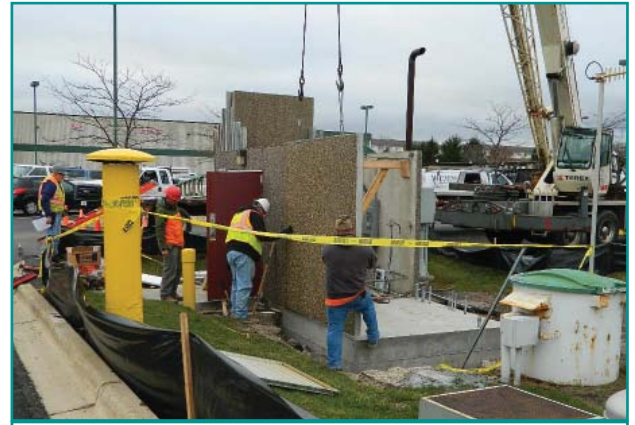
Lift Station Retrofit at 521 North Avenue
