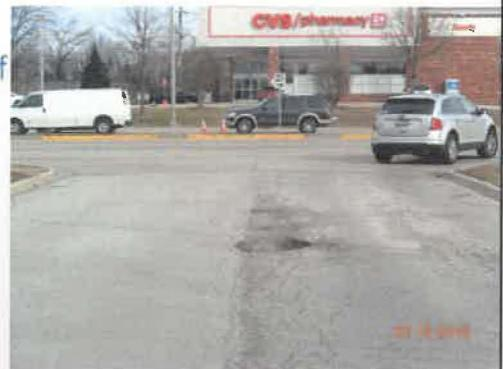
Code Enforcement notified this private property owner of the over 4 foot long by 2 ½ foot wide pothole in the access drive. Patch was applied in the hole within 3 days.
