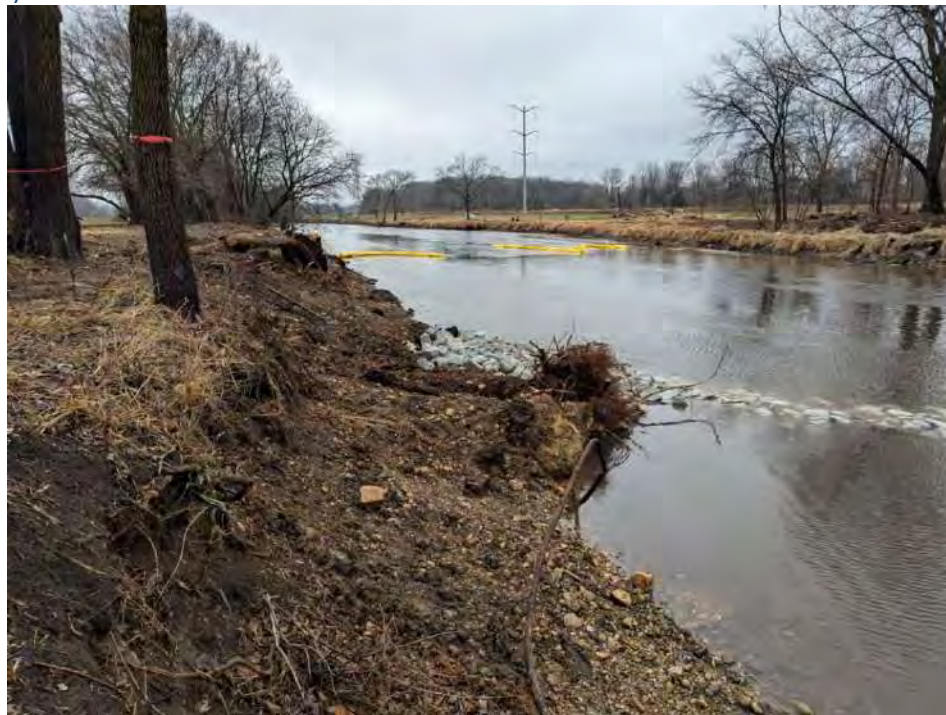
Plate 27. Photographs of rootwads and stream barbs on the east side of the Lower DuPage River (Winter 2025)
