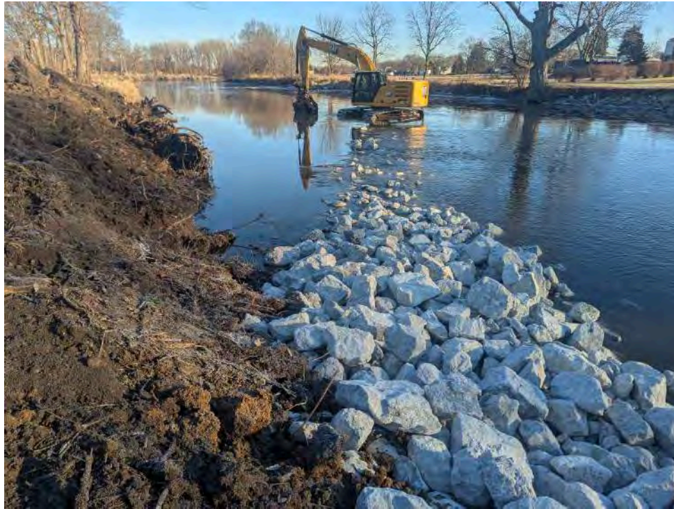
Plate 25. Photograph of a brush box being installed on the east side of the Lower DuPage River (Winter 2025)
