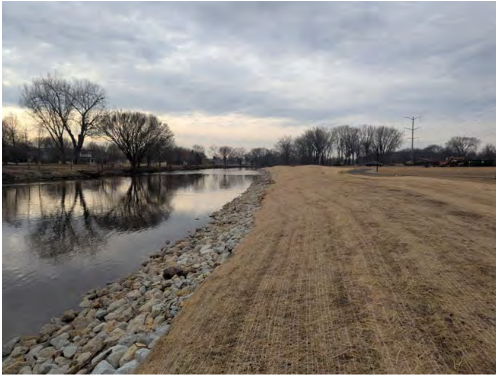
Plate 20. Photograph of the completed boulder toe with seed and erosion control blanket on the west side of the Lower DuPage River (Winter 2025)
