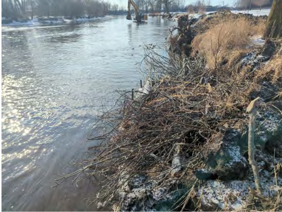
Plate 27. Photographs of rootwads and stream barbs on the east side of the Lower DuPage River (Winter 2025)
