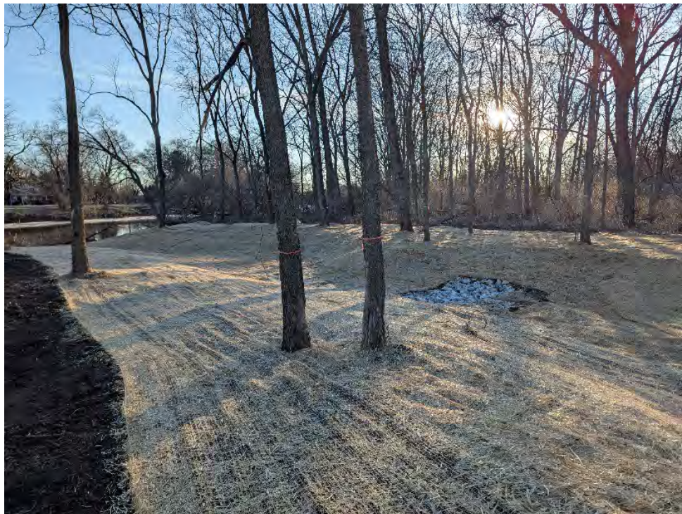
Plate 32. Photograph of Swale 5 after being seeded and stabilized with erosion control blanket (Winter 2025)
