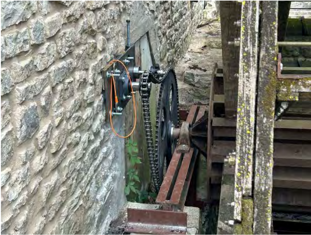
Plate 15. Photograph of the gear and chains associated with the motor during installation on the Graue Mill waterwheel
